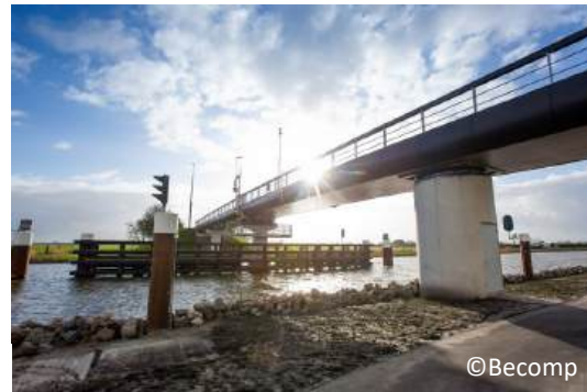
Ritsumasyl-Bridge (NL) 30to of Bio-Composite instead of 400to steel/concrete
